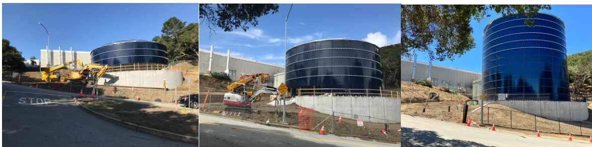
Water Supply Tank Replacement
