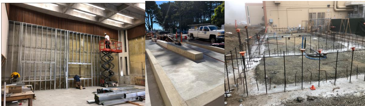
Building 1 Social Science and Creative Arts Building Facelift
